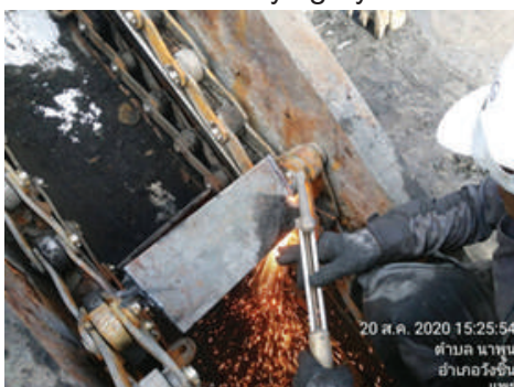
Corrective maintenance of ash conveying system
