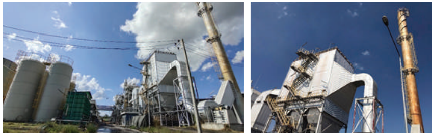
Picture of air pollution treatment with electrostatic precipitator technology (ESP)
