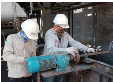
Corrective maintenance of ash conveying system
